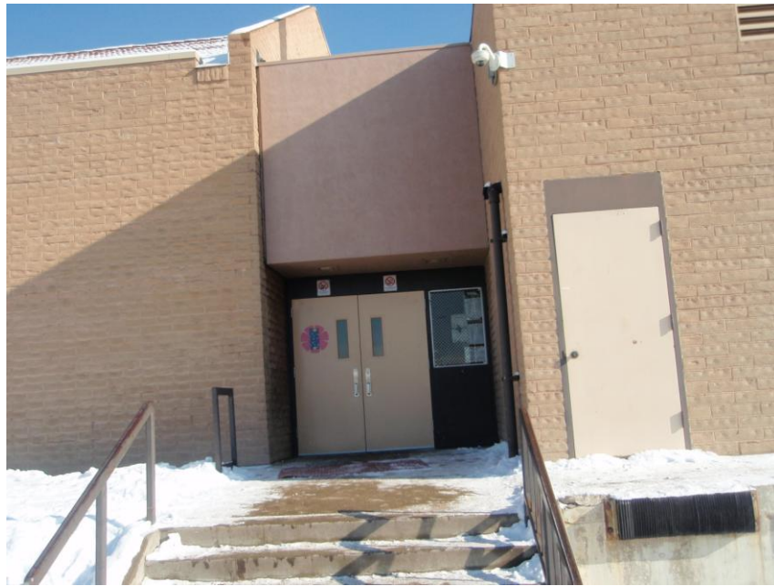
Current west entrance
